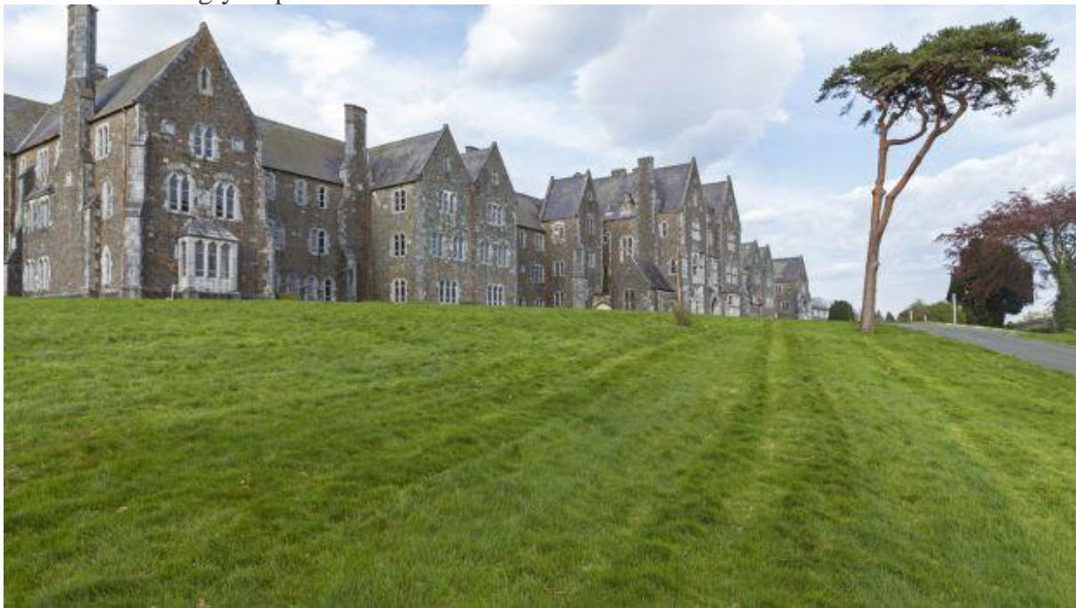
St Finan's Hospital, Killarney, Co Kerry, opened in 1852 in the aftermath of the Famine. Photograph: David Killeen
